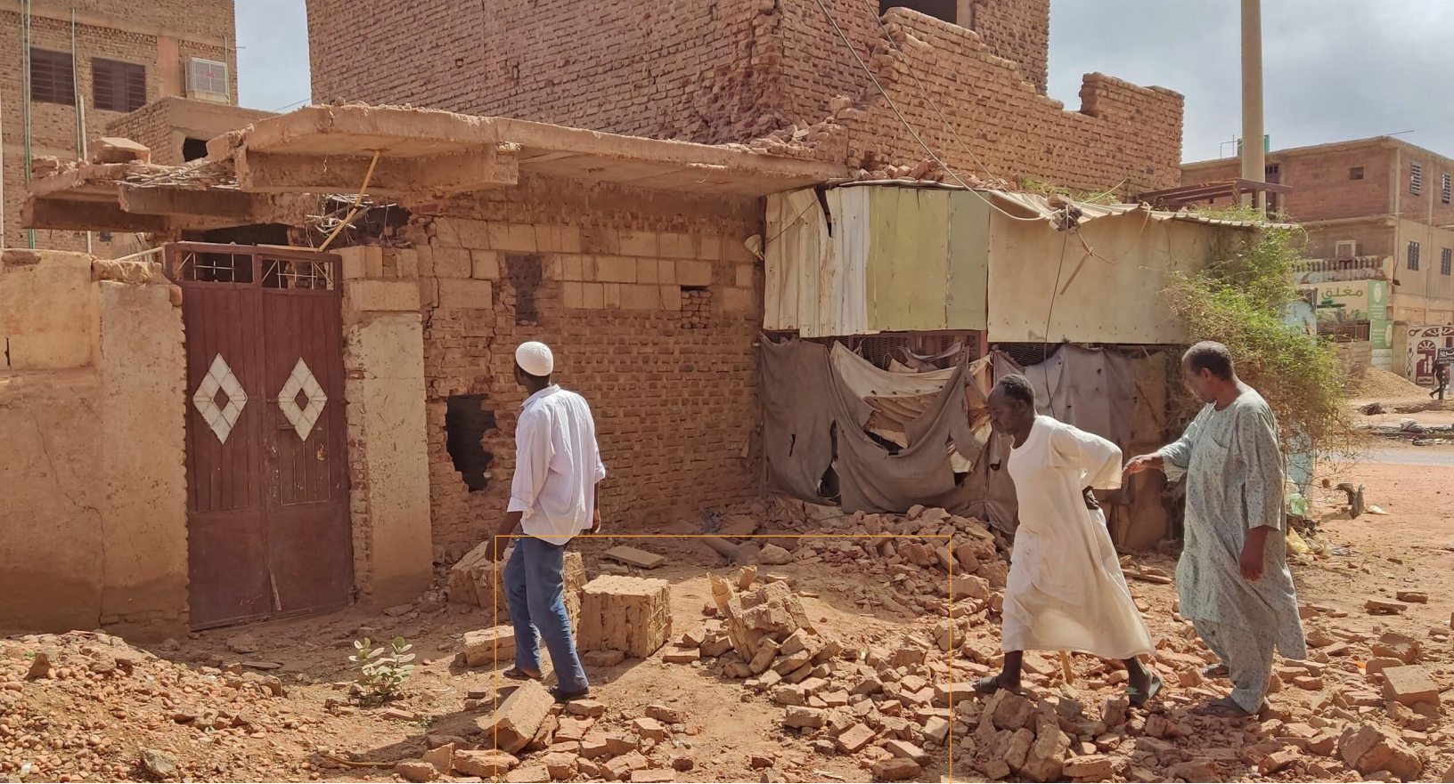
People check a damaged house in southern Khartoum, Sudan on June 12, 2023. (Photo by AFP via Getty Images)
